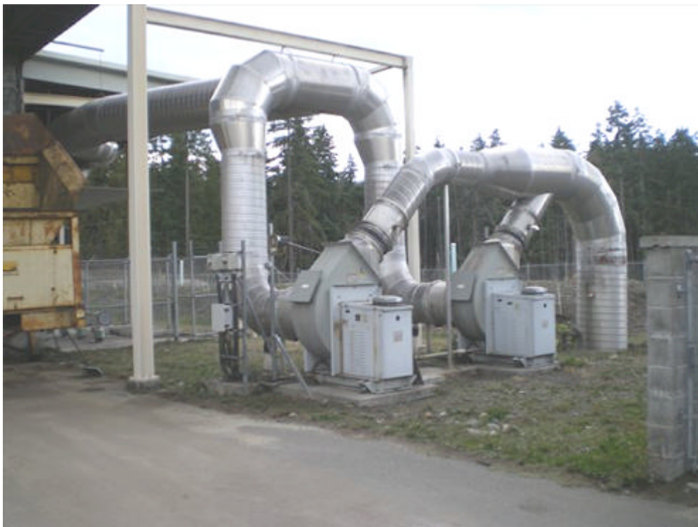
Air handler and exhaust ductwork supply to biofilter, Bevan Road, Cumberland
